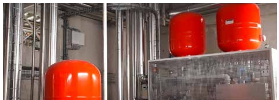
Hot and cold water distribution system for the equipment used to distribute liquefied chocolate.
